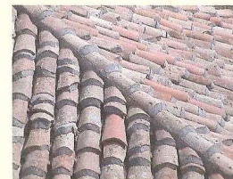
Clay tile hipped roof and ridge.
