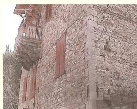
limestone walls with wooden batten and quoins.
