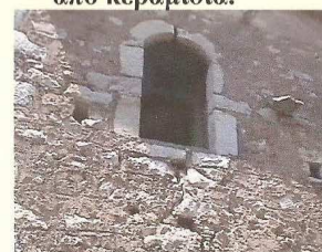
Small arched openings with surround cut stone decoration.
